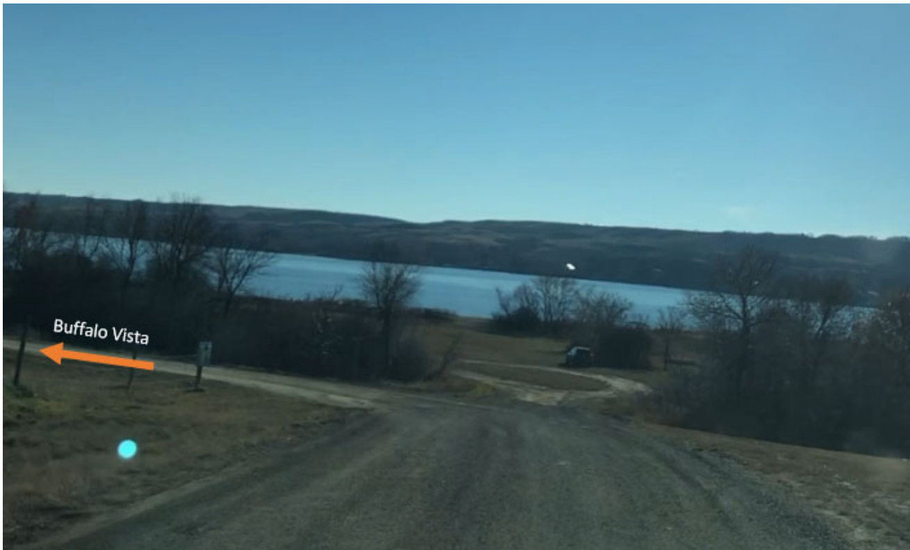
Figure 2: Access Road into Buffalo Vista – Looking South on Daniel Drive
