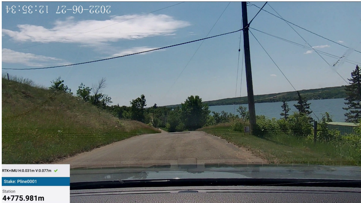
Figure 5 - Location of a low overhead power line, recommended that low clearance warning signs installed in both directions
