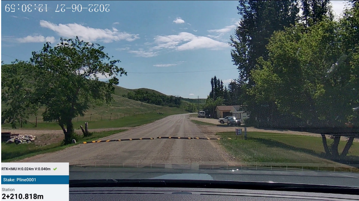
Figure 1 - Temporary speed bump that is recommended to be replaced by a permanent speed bump
